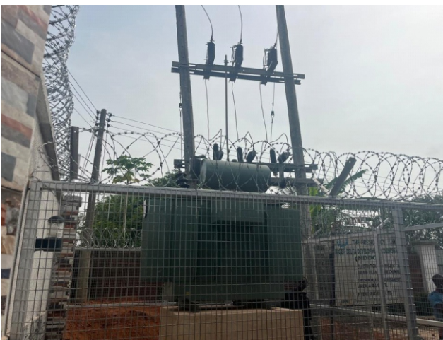
The newly installed 500 KVA transformer at Iyiocha
