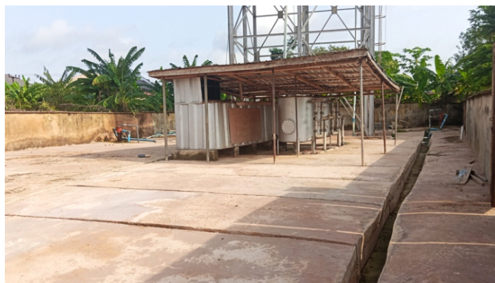
Concrete flooring at water tank facility
